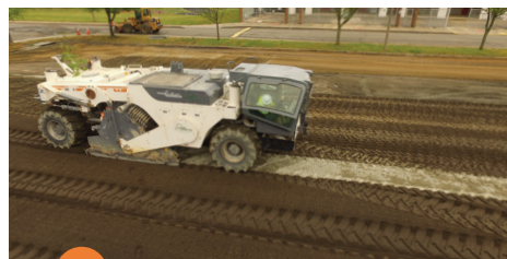
4 Full-Depth Reclamation (FDR) in action.
