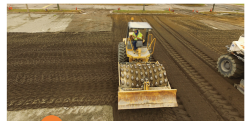
5 Padfoot roller provides deep compaction.
