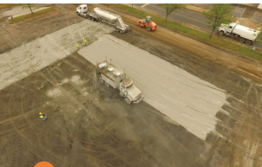
3 Portland Cement is spread on the pulverized and re-graded mixture.
