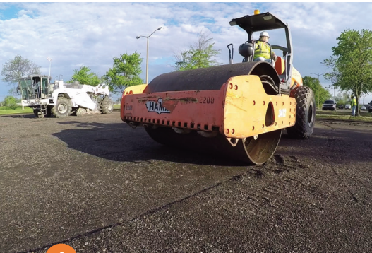
6 Reclaimed area rolled and compacted.
