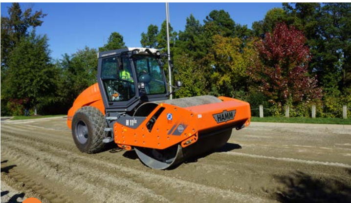
6 Initial compaction with roller
