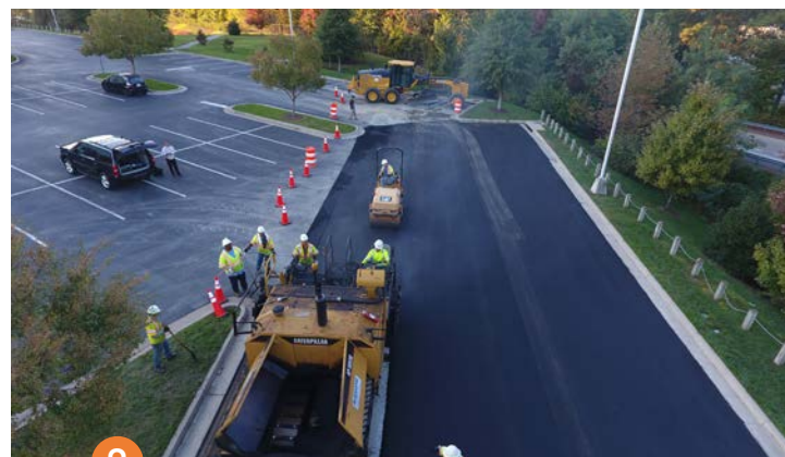
9 The last pull on the 2.5 inch overlay
